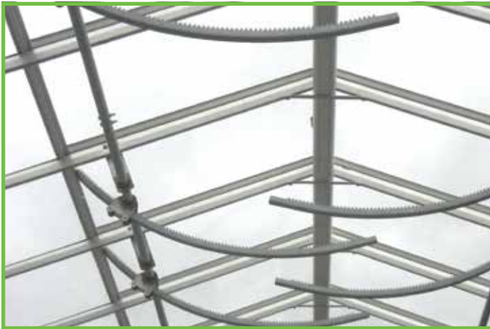
Ridder Curved Steel Rack Arm at Double Roof Vent
